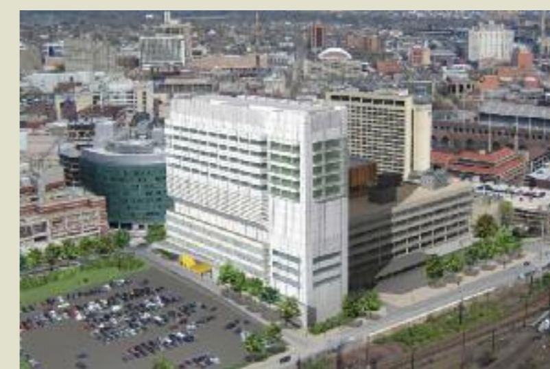
Penn's Translational Research Building will be one of the first anywhere to be physically integrated with patient care facilities.
